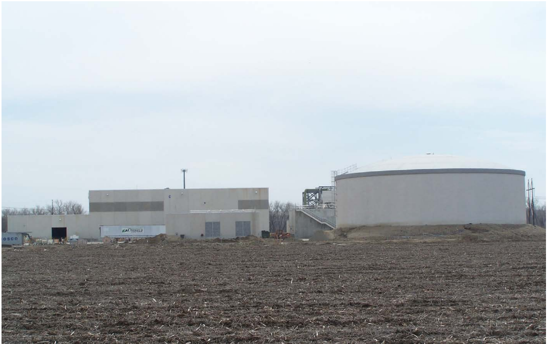
COUNCIL POINT WATER PURIFICATION PLANT UNDER CONSTRUCTION 2012
